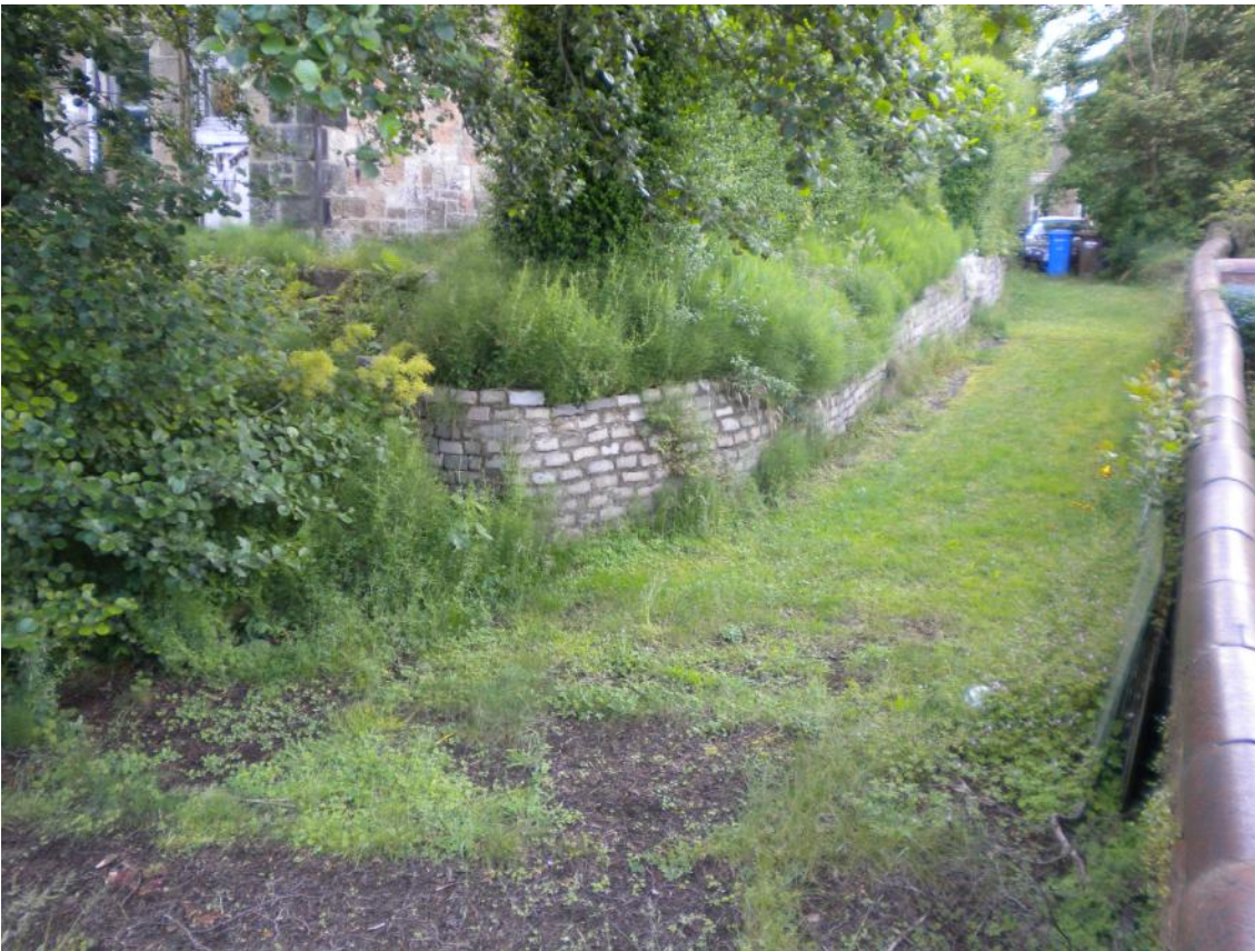
Fig.2. Newark Drive - Grassed over concrete driveway.
